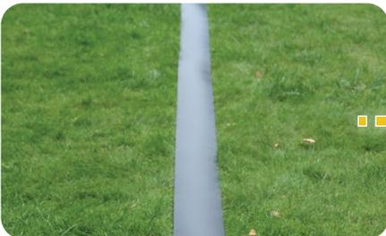
Uncoil the B-Edge Pro (XL) by putting a weight at the ends during mild ambient temperature, preferably in the sun. This allows the edge to flatten.
