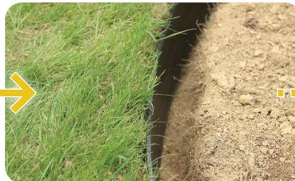
Create a ditch to separate two area's by the B-Edge Pro (XL) and insert evenly, allow enough to prevent soil, gravel or mulch to easily drop into the adjacent area. As shown in (3) install 20 cm long steel nail for additional hold, if required (not supplied)
